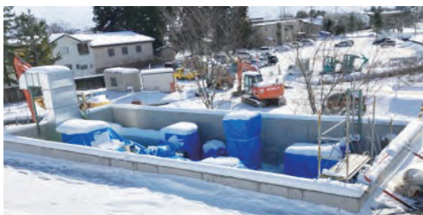
図9 現地施工状況 Fig.9 On-site construction status
