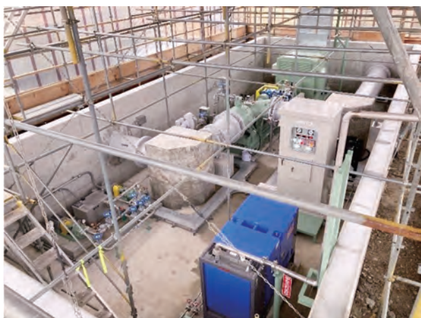
図11 現地据付状況 Fig.11 On-site installation status
