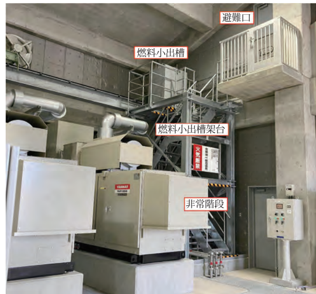
図6 非常階段付き燃料小出槽架台 Fig.6 View of the emergency staircase
