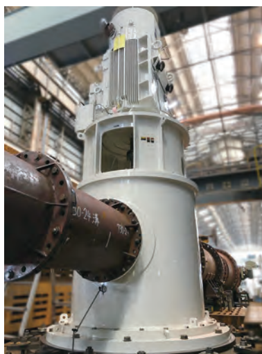
図8 温水ポンプ据付外観 Fig. 8 Installation view of Hotwell pump
