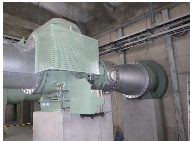
図9 低圧力損失形逆止弁外観 Fig.9 View of- low pressure loss check valve
