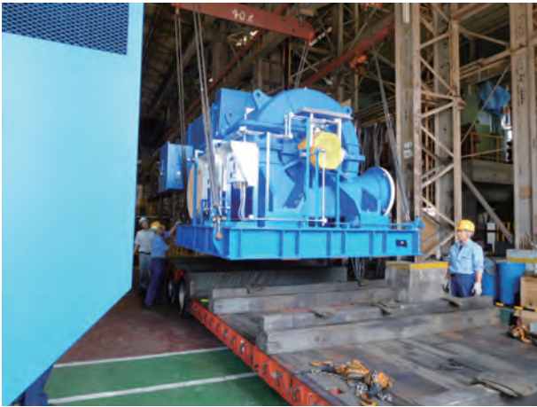
図5 ブロワ吊り状態 Fig.5 View of blower lifting
