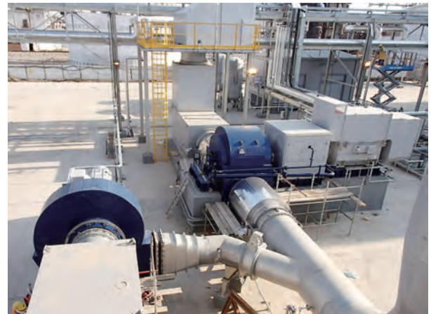
図9 ブロワ現地据付状態 Fig.9 View of blower on site
