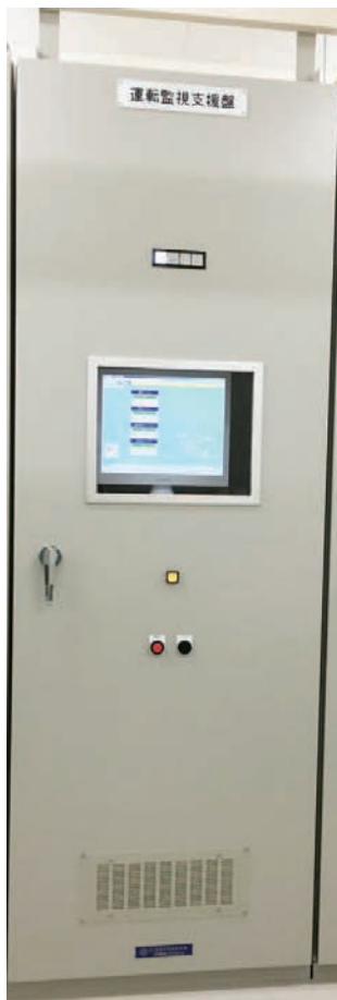
図6 運転監視支援盤外観 (各トンネル) Fig.6 View of operation monitoring support panel
