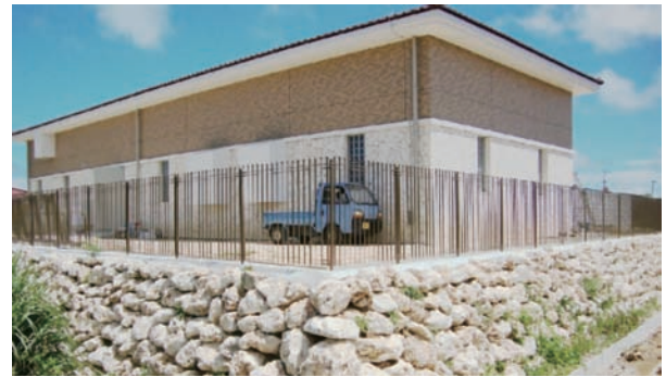
図4 余多揚水機場外観 Fig.4 View of Amata irrigation station
