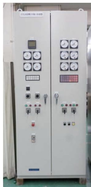
図5 動力制御盤 Fig.5 Power control panel
