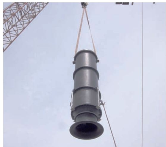
図5 現地写真 Fig.5 Lift up of pump assembly
