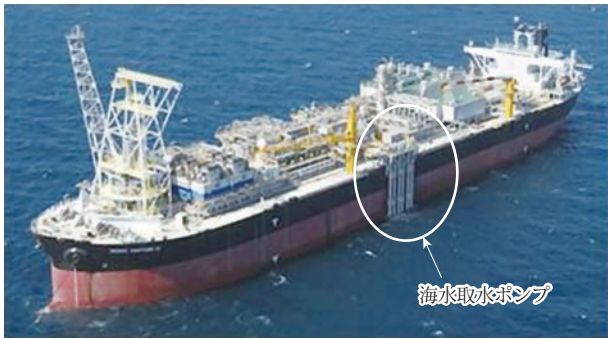
図2 FPSO外観 (1) Fig.2 View of FPSO
