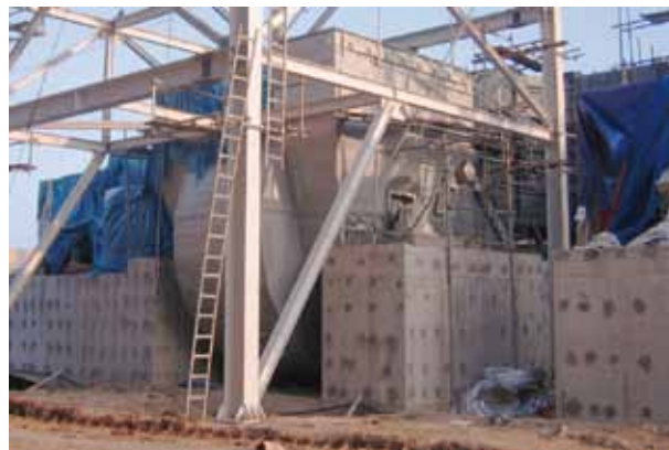
図10 IDF据付状態 Fig.10 Installation at site
