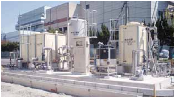
図6 除鉄・除マンガン装置据付外観 Fig.6 View of iron and manganese removal products
