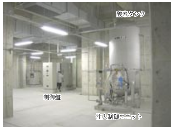
図12 酸素タンクと制御盤 Fig.12 View of oxygen tank and control panel
