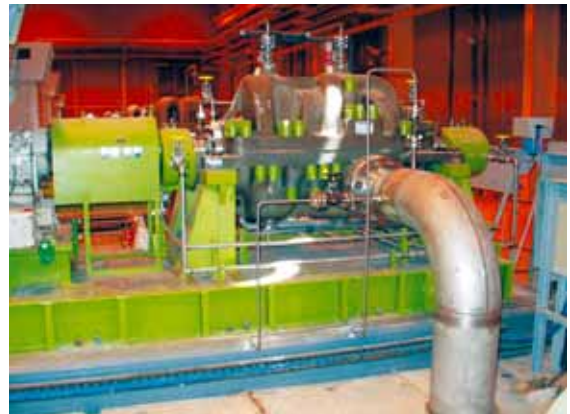
図6 現地稼働中のポンプ Fig. 6 View of high pressure pump at site
