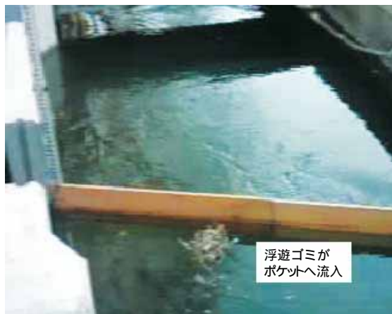
図10 ポケットへの浮遊ゴミ流れ Fig.10 Flow of float rubbish into pocket
