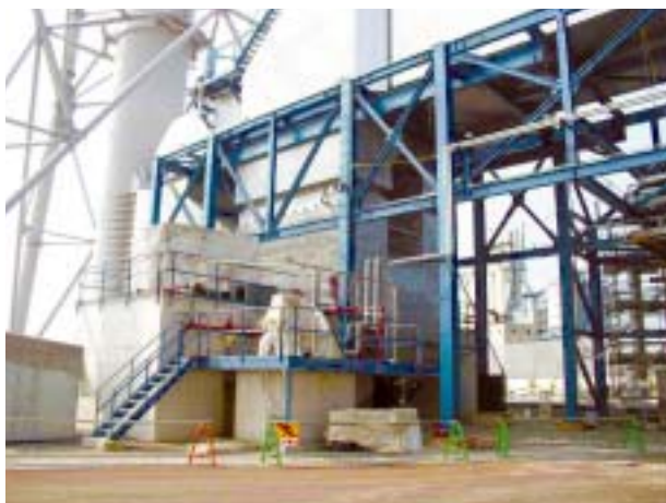
図6 BUF全景 Fig. 6 View of BUF at site
