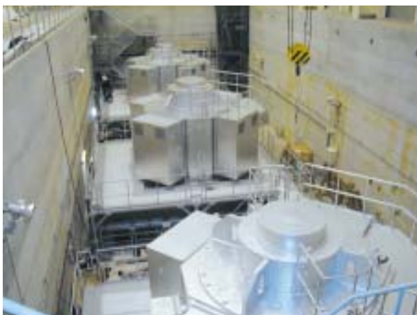
図1 据付外観 Fig. 1 View of installation
